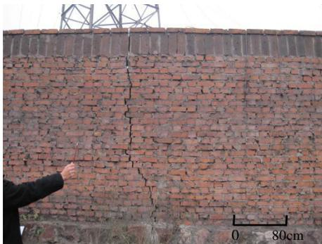
Figure 4 housing cracks
